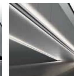
LED cove lighting Side and soffit cladding
