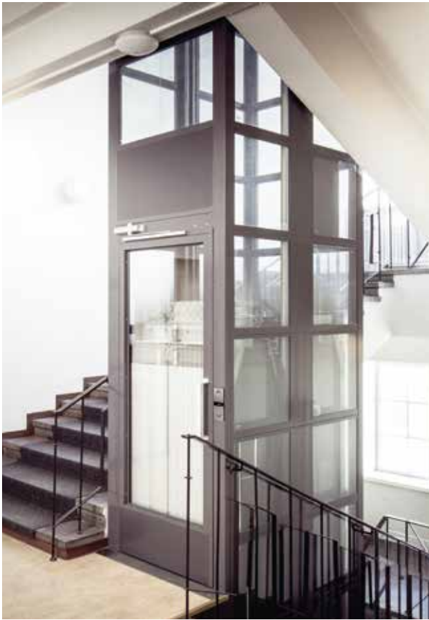
The KONE ProSpace lift shaft is self-supporting, so it puts no stress on the building walls.
